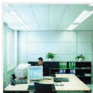
Fig. 52: In the morning, no light is needed from the row of luminaires near the window.
