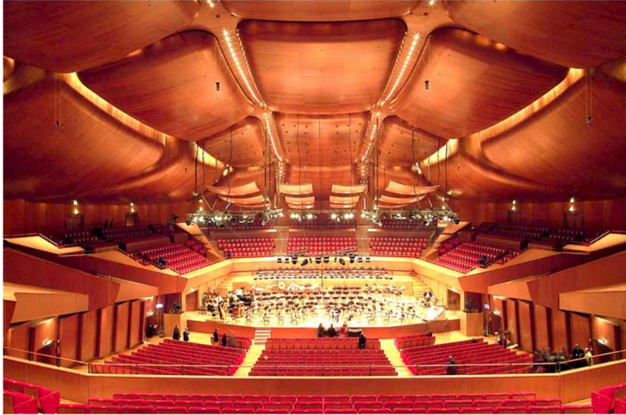
Fig. 1. The Santa Cecilia Hall as seen from the front rows of the main rear gallery (courtesy Photo Maggi). Note coffered ceiling designed to reflect the sound diffusively, with no privileged direction; the curved reflector panels above the orchestra that can be oriented in different ways; lateral cavities created by the presence of the side galleries; curvature of the upper parts of the walls and tilted panels coating the lower parts: all these elements contribute to minimizing specular reflections, and to create a diffuse sound field.
